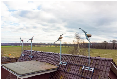
SkyWind NG turbines installed on a residential roof near Hamburg (Germany). Photo Credit: SkyWind Energy
